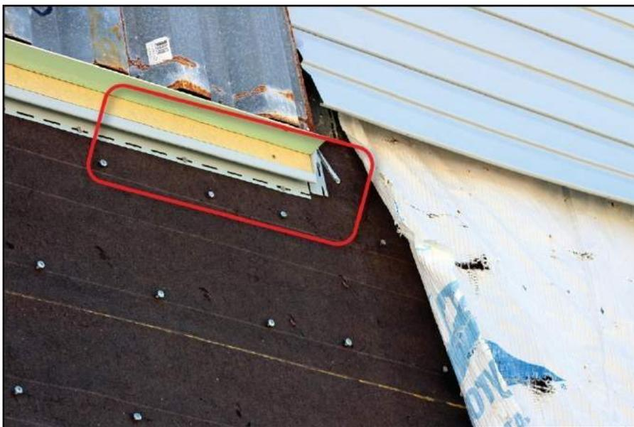
Vinyl Siding Institute (VSI) conducted several recent post-hurricane analyses and noted the need to have these requirements added to the IRC to avoid future cladding system failures. An example showing failure from Hurricane Irma that resulted from improper installation is shown below.
