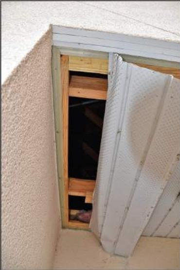
Another non-residential soffit failure at roof overhang is documented at the Bay County Courthouse addition (MAT Report Figure 5-110, shown below) where repairs to interior damages caused by the soffit breach, roof membrane damage, and flashing deficiencies at the ridge and hips were estimated to cost \$477,000.
