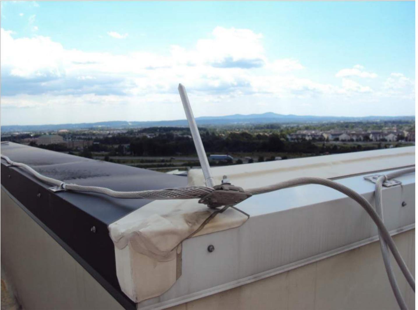
Due to the installation of the Lightning Protection System components there may be certain details which require additional hot air welded patches installed under cable splices, frayed cable, and specific connections that could abrade the membrane. Hot air welded patches will provide sufficient protection to the field membrane from abrasion. Pictures below show examples of areas where additional hot air welded patches would be required.
