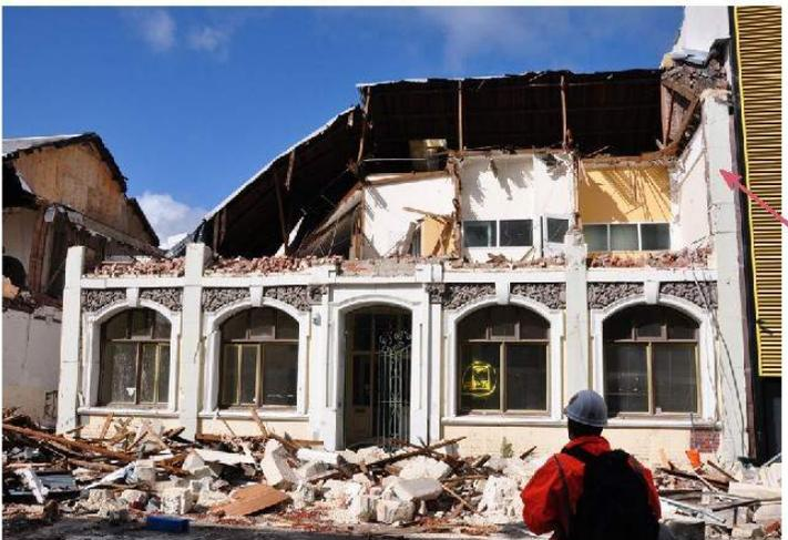
Photo of damage to masonry building in Christchurch.
